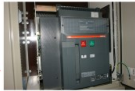
1600A 4 Pole Air Circuit Breaker
